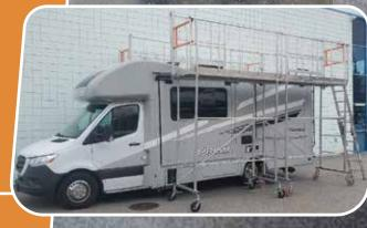
ROOFTOP HANDRAILS PIVOT 90 DEGREES FOR DRIVE IN-DRIVE OUT
